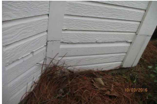
Siding damage on each side of the breakfast nook.
