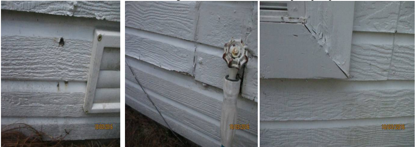
Nail holes, siding and window trim between pool pumps and nook.
