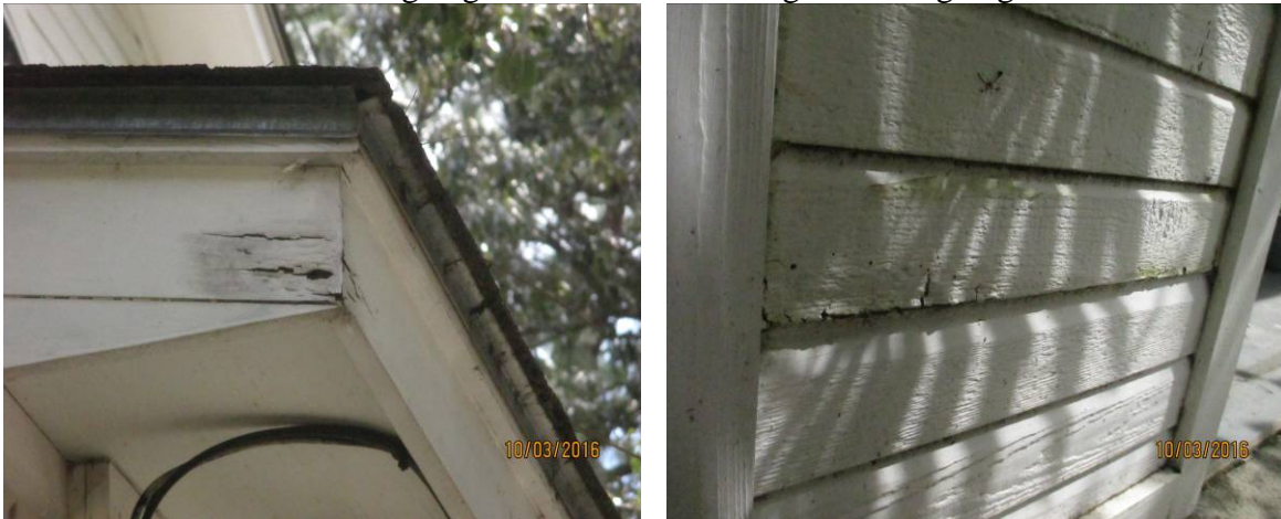
Front corner garage end fascia and siding between garage doors
