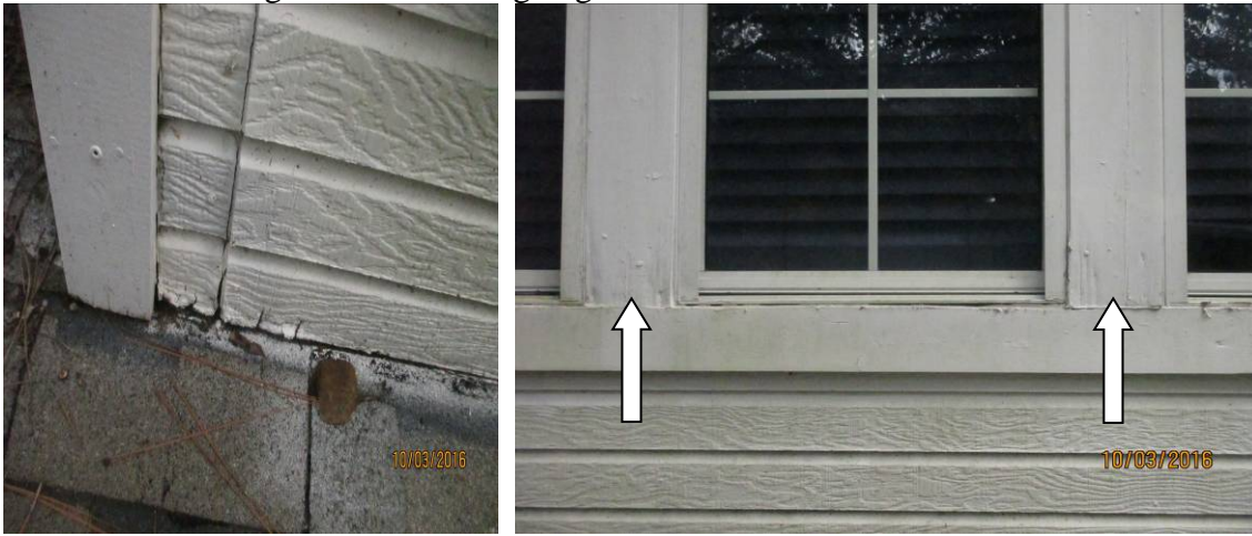
Siding and trim above garage on second level
